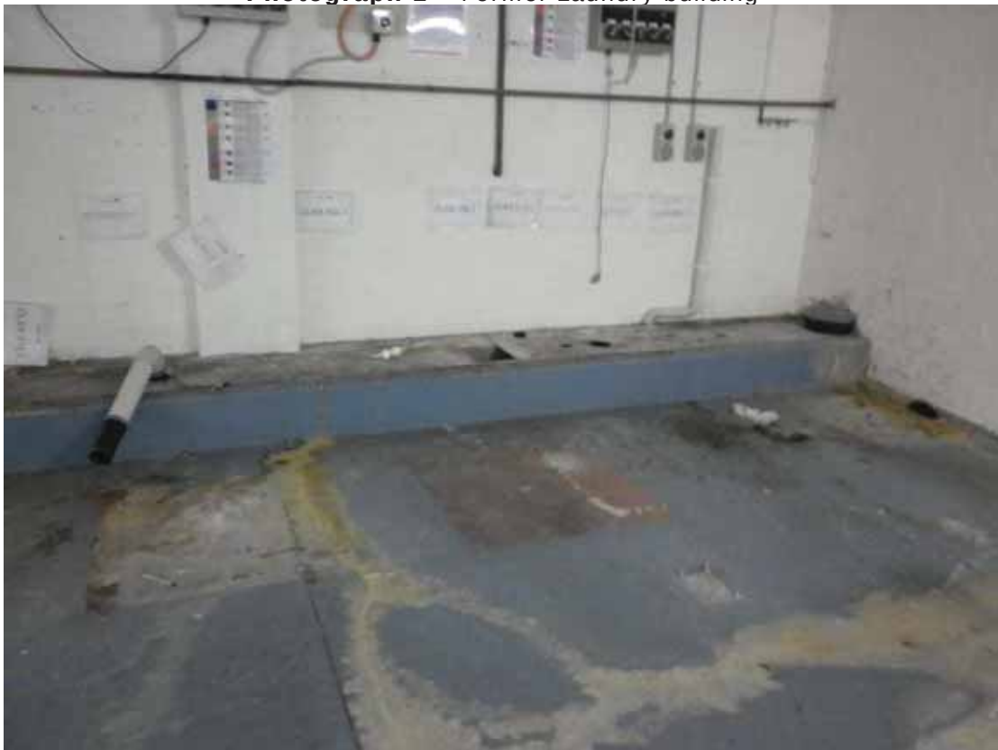
Photograph 2 – Inside the laundry building
