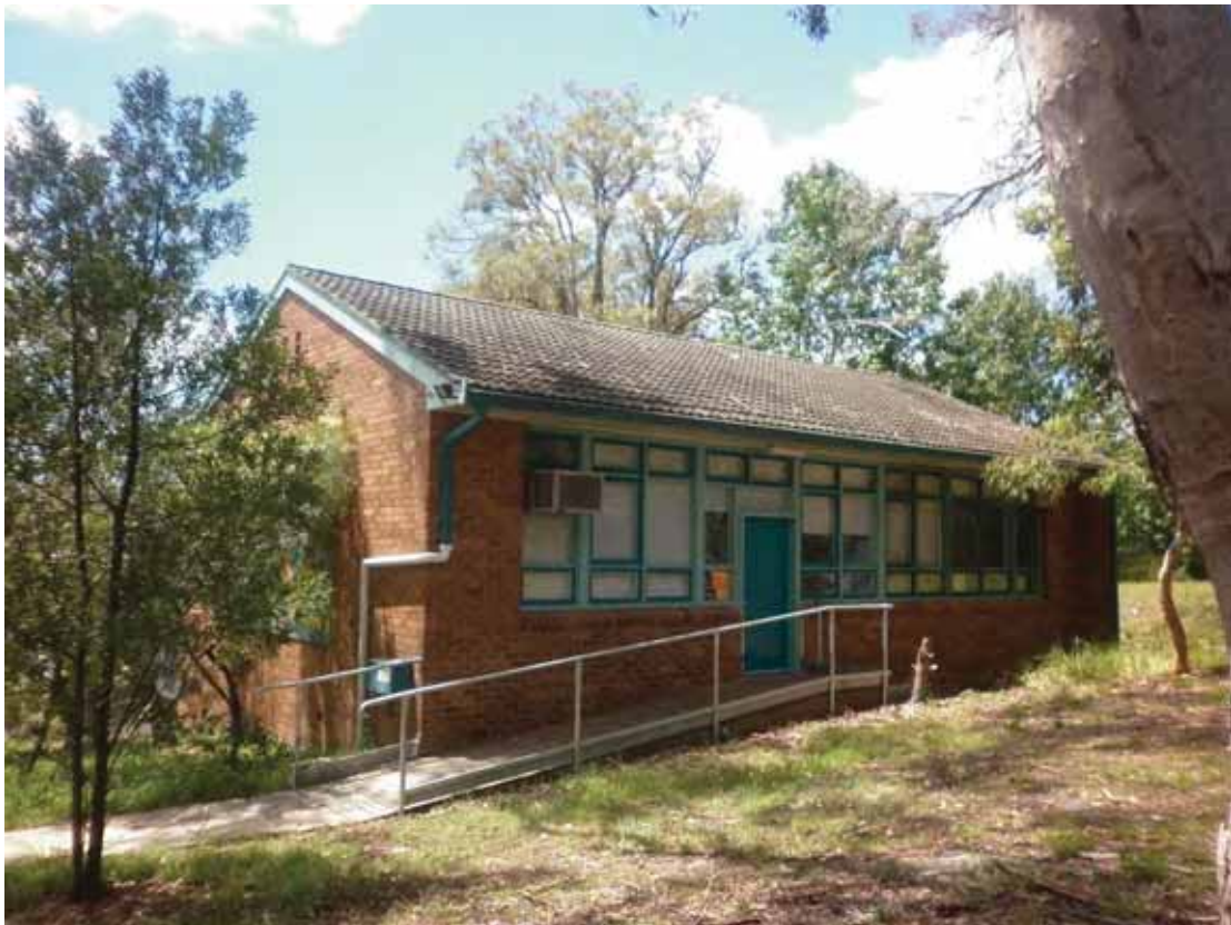
Photograph 26 – View looking south at the Former School
