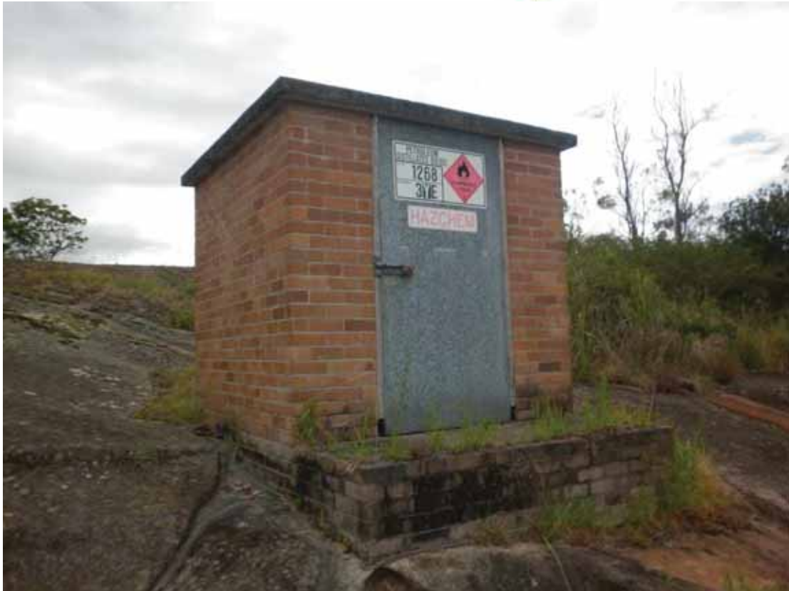
Photograph 7 – Disused AST on mainland shed
