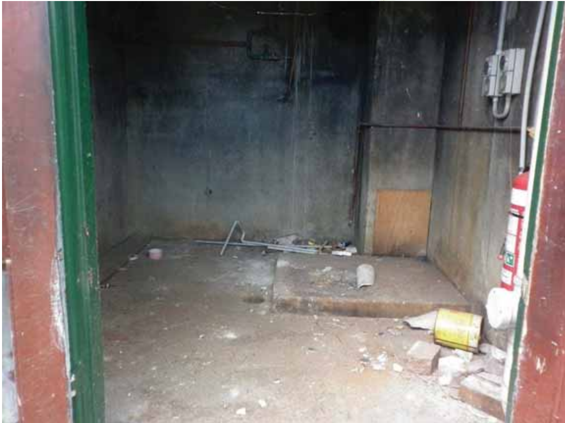
Photograph 11 – Former Boiler Room on Peat Island
