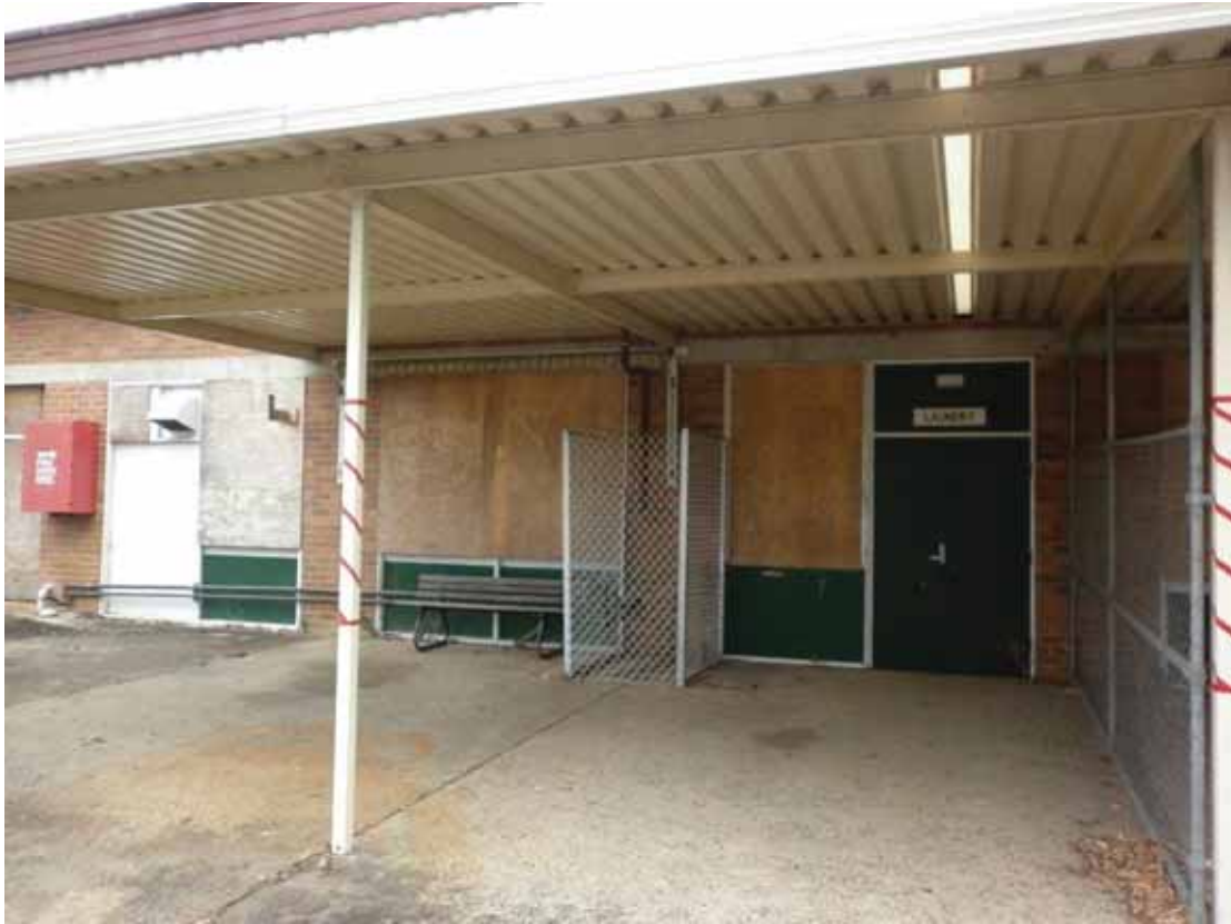
Photograph 1 – Former Laundry building
