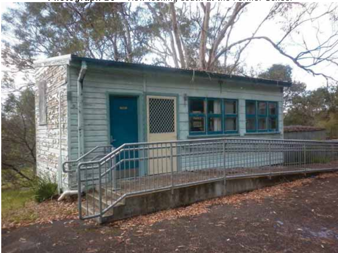
Photograph 27 – View looking south at the Former School
