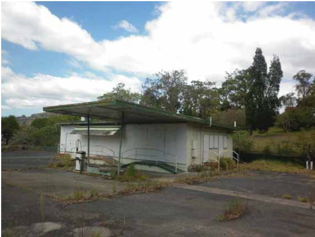
Photograph 23 – View looking west at the Former Service Station
