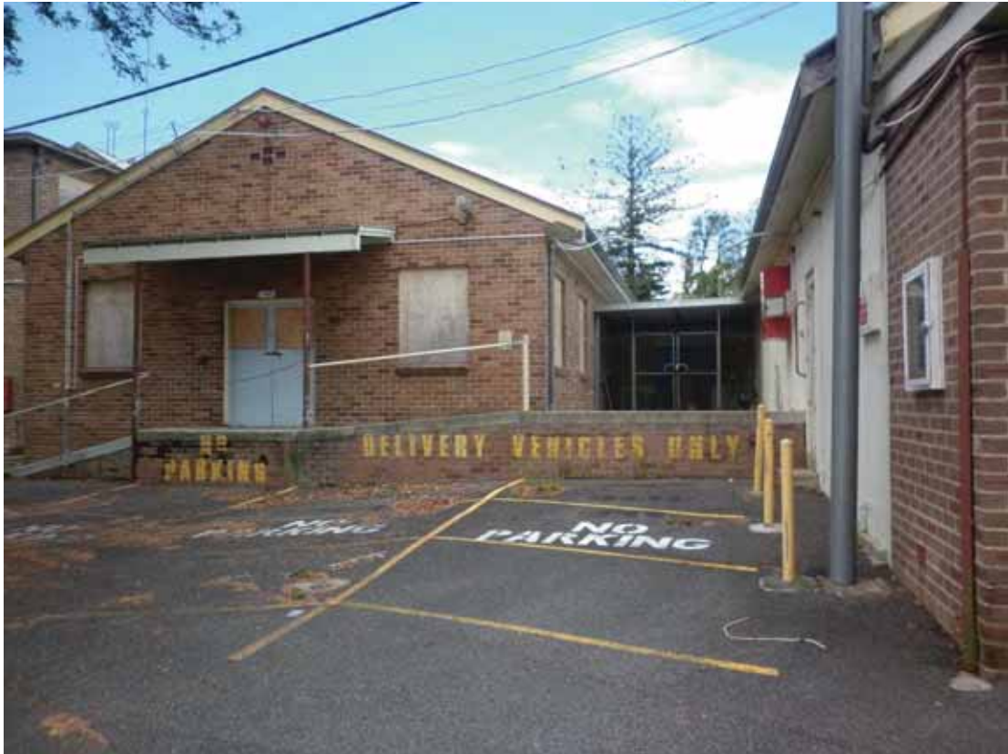
Photograph 15 – View looking west at entrance to site
