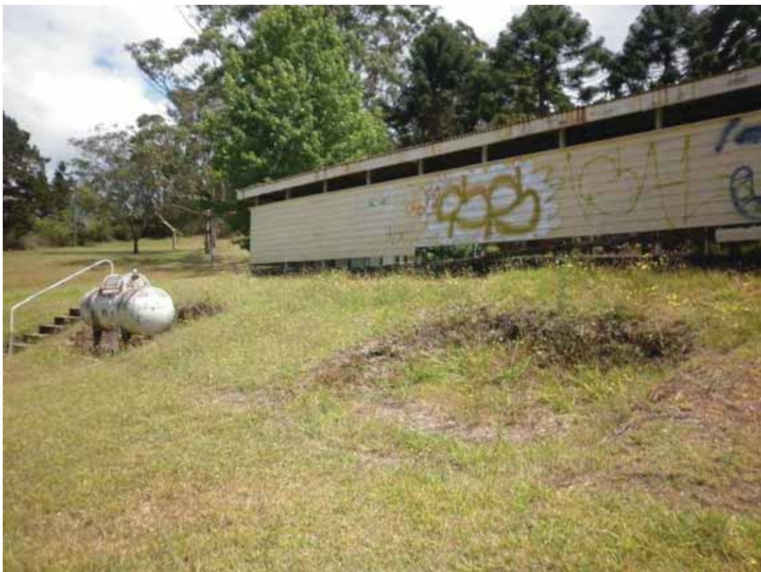
Photograph 20 – LPG Gas tank adjacent to the accommodation
