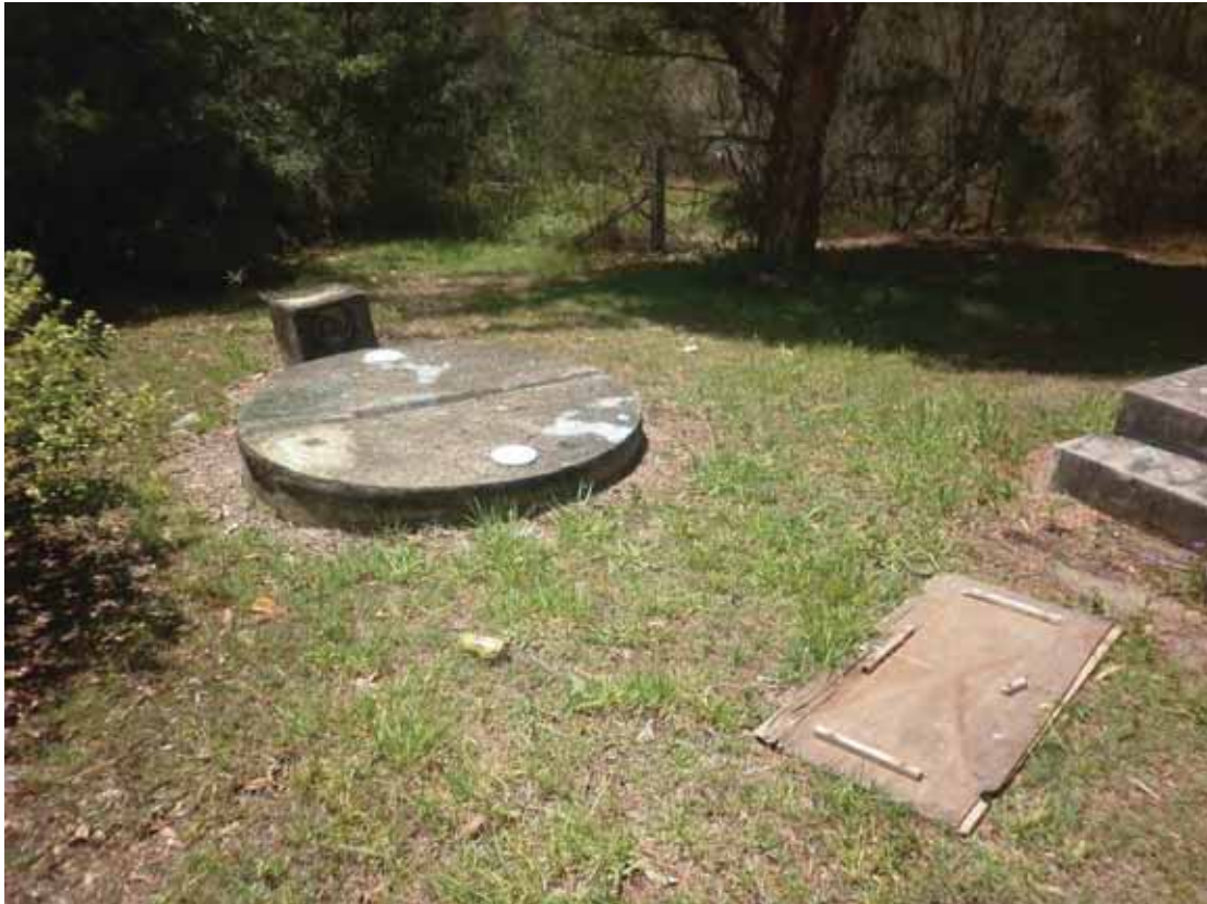
Photograph 28 – View looking south at the septic tank
